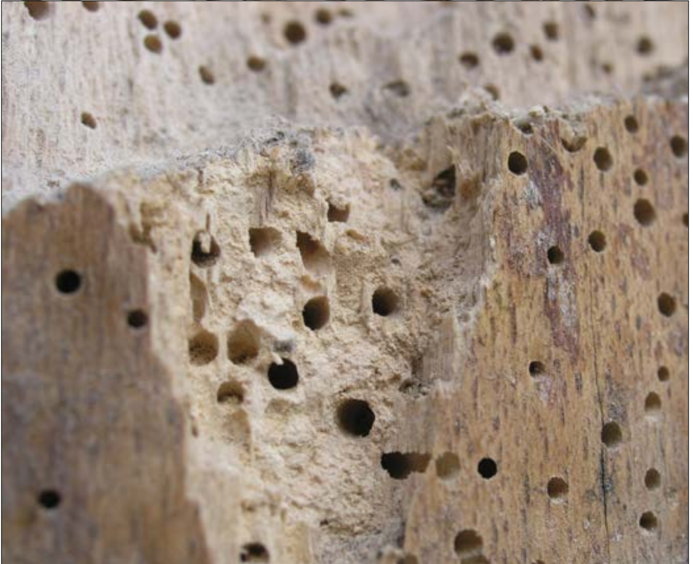
Evidence of woodworm damage are exterior holes in the wood and sawdust on the floor.
