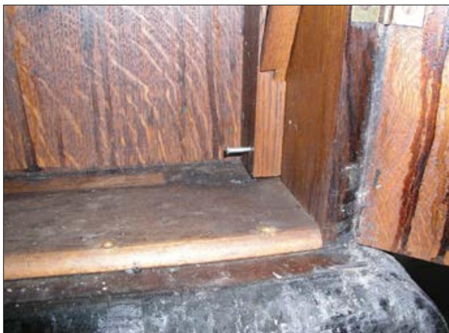
A detail shot showing the damage caused to the base by the fire.
