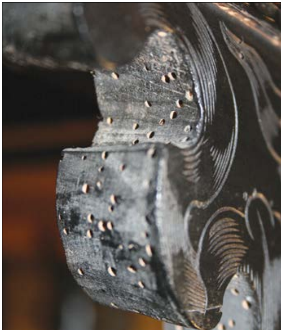
Damage from woodworms can be quite extensive.
