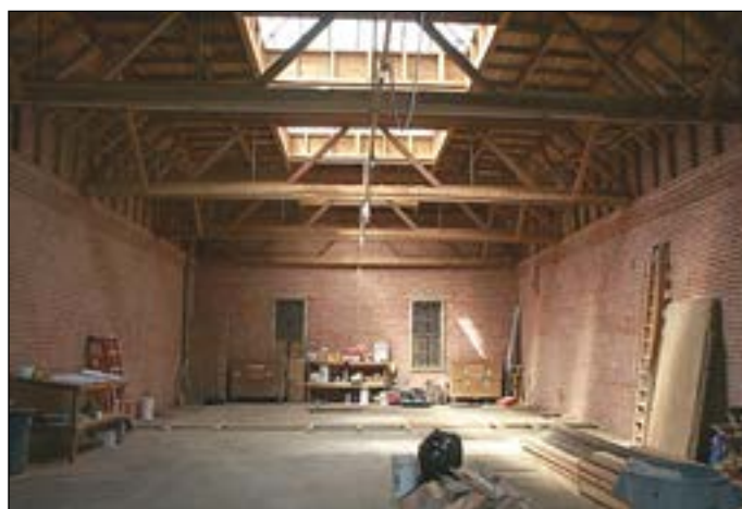
The interior of the building after sand blasting.
