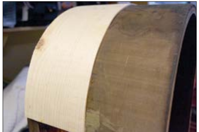
The curved top of the case, showing a pine wood substrate epoxied to the underlying wood.
