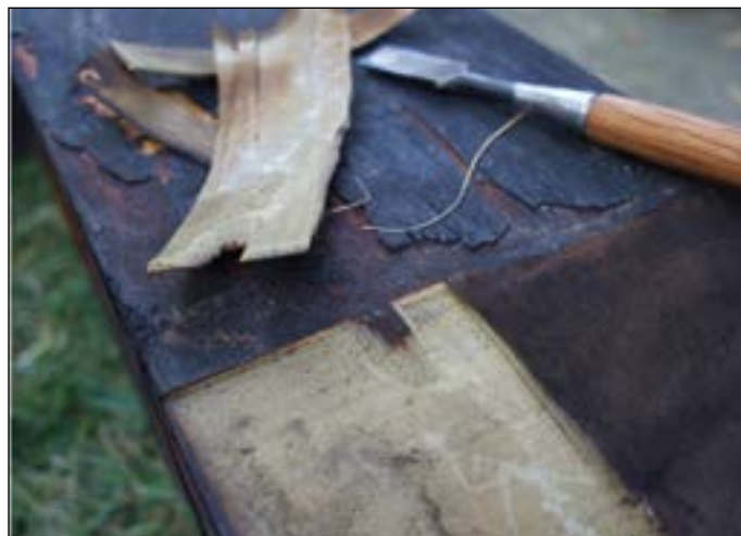
Removing the burned wood with a chisel.
