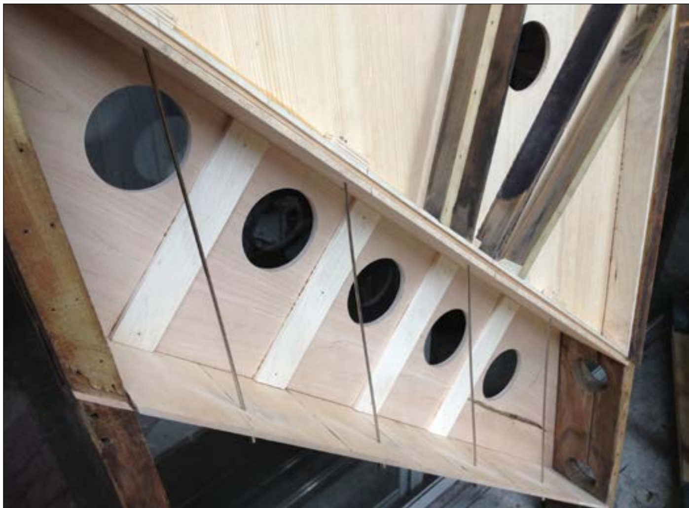
The remade sound box in maple, strengthened by 1/8" steel rods installed vertically to help support the fret board.
